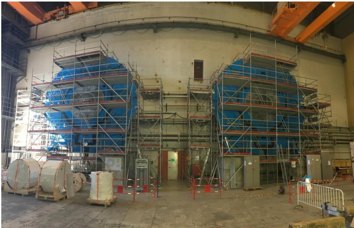
**Figure 2: Two views of the shielding disk (NJD) which will support the chambers, in b191, shown with and without scaffolding, and with services routed around its periphery.**
